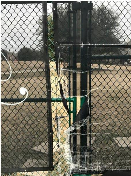
**Replace broken zipties quickly.** When too many zipties holding the screen have broken and the windscreen starts to whip against the fence, it can be damaged beyond repair in a few hours. Damage caused by wind force in this manner is not covered under warranty.
